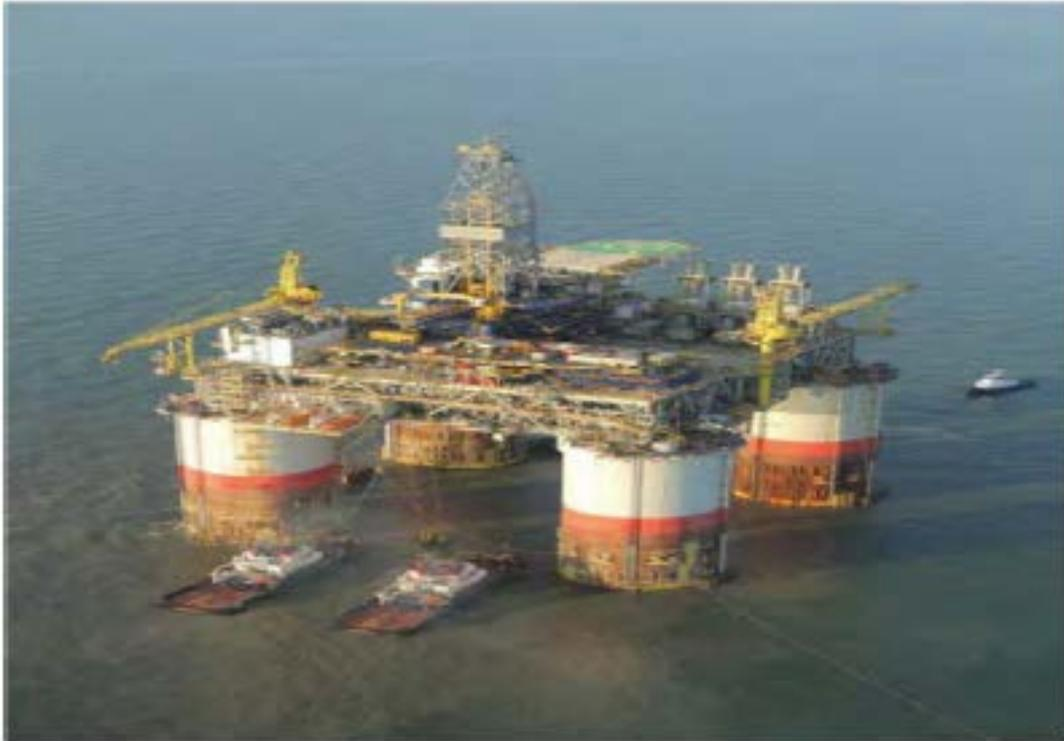
The platform would be kept stationary by sixteen steel tendons attached to pilings driven into the seafloor. These tendons were critical to the floating platform's stability.
